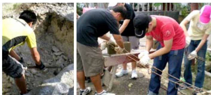
Digging the septic tank Tying of wires
