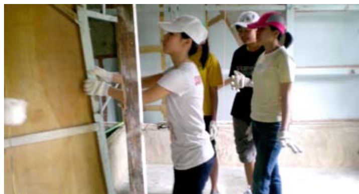
Removing all the nails on the wooden doors and walls
